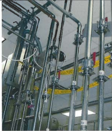
Welding of utility connections
